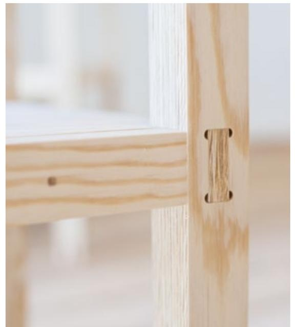
Our Joint Detail, 36mm profile made up from 3x12mm laminated Pine plywood
